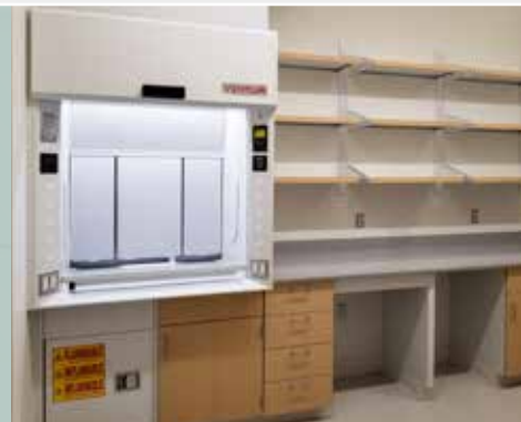
Vertical Rising Sash with Automatic Sash Operator
